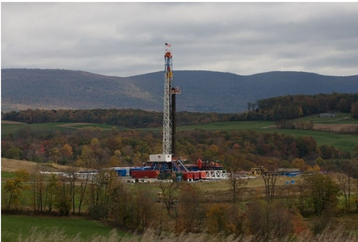
A typical Marcellus gas well site (Tom Murphy, Lycoming County Cooperative Extension).
